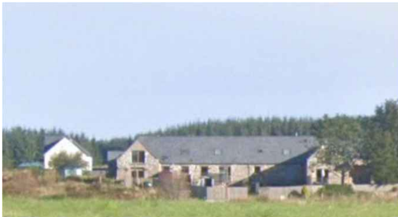
Bogriffie Steading conversion
