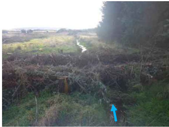
Fig. 4: View downstream of the lower section of the Channel 2. Brash bridge made by the forestry for extraction purposes.
